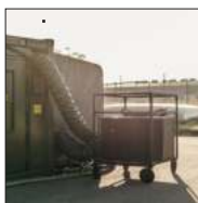
Militarized HVAC unit with ducting
