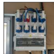
Distribution board & fittings for single and/ or 3 phase integration
